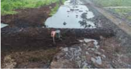
Figure 3-12a (left): Compacted peat dam constructed in series of 5 along the 20+ metre-wide canal along the western side of the Tahura OKI (buffer zone of Berbak NP); these were constructed in the wet season Jan-Feb 2018 and were functioning well after 1 year (Photo courtesy of Mott MacDonald).
