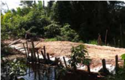
Figure 3-16: An Earth-fill Block made of wood, soil bags and earth fill in a medium-width canal
