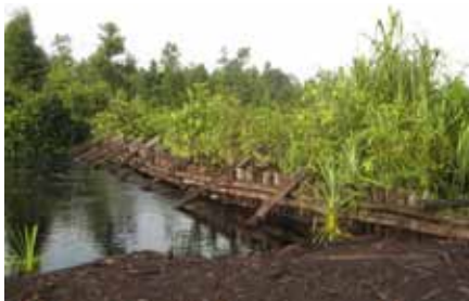
Figure 3-21: Multilayer block constructed in 2005 in abandoned primary inlet canal of the Mega Rice project Block AB in Central Kalimantan. Block is 30m wide and canal is 10 m deep. Main posts are 12-15 m long and inserted to mineral layer below the peat. 25,000 sand bags (wrapped in two large geotextile sheets) were used in the construction completed by hand by a team of nearly 100 workers over one month. (Photo courtesy of Alue Dohong)
