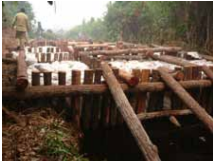
Figure 3-20: Plank Block in small drain. (Photo courtesy of Alue Dohong)
