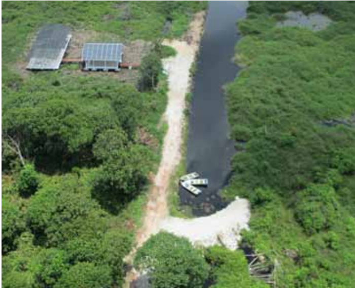
Figure 3-18b: Same rock-fill dam in 2014, one year after construction
