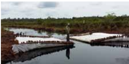
Figure 3-23: Geotextile wrapping of large block and central spillway to prevent erosion.
