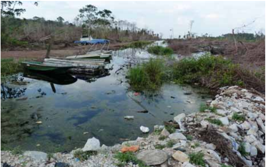
Figure 3-18a: Rock-fill dam in large canal in early late 2012, 2 months after construction
