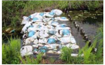
Figure 3-15: Sandbag block in large canal.
