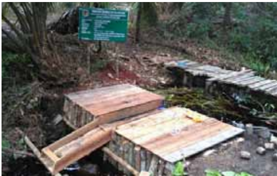
Figure 3-19 (left): Timber Box Block for small canal (Source: Ministry of Environment and Forestry, Indonesia)
