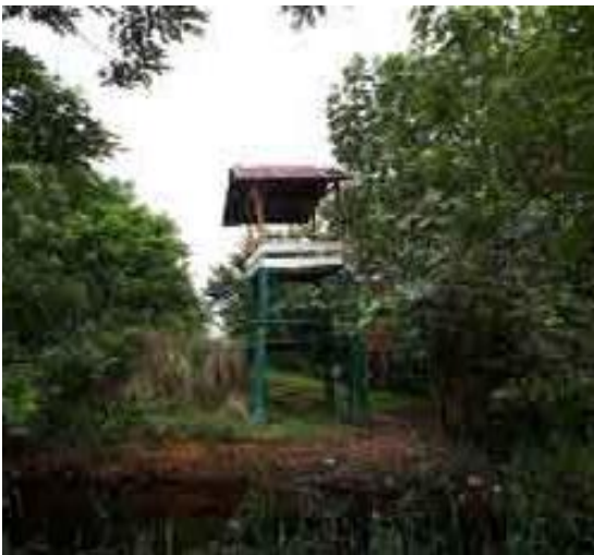
Location: Tower Monitor of MGE 2.
