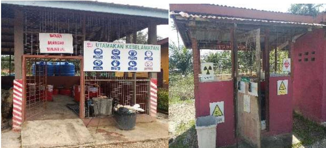
Schedule Waste Storage Area
