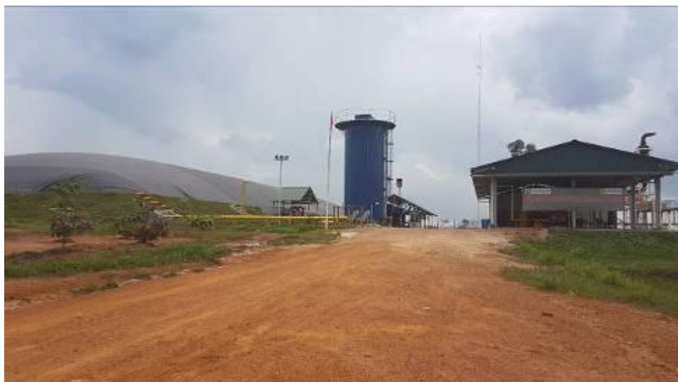
Biogas Plant at Tengkalat Mill
