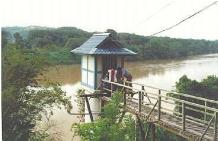
Figure A4.8: A Water Elevation Telemetry Station installed at Sg Kuantan (DID Malaysia)
