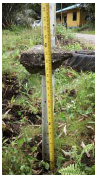
Figure A3.1: Example of subsidence pole installed
