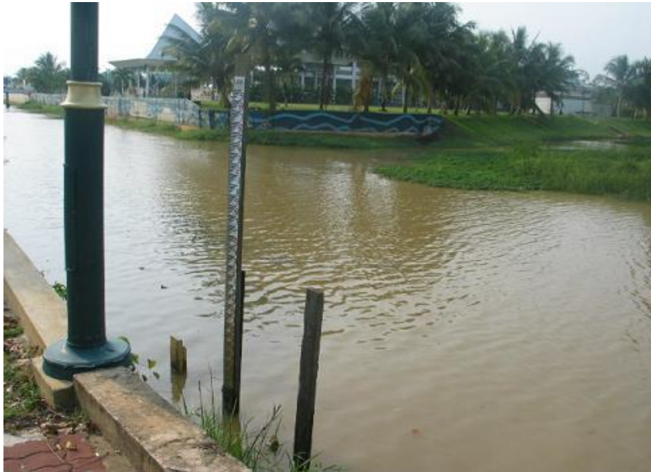
Figure A4.3: A staff gauge installed at Sg. Pahang (DID Malaysia)
