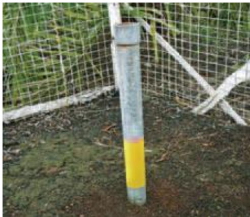
Figure A3.2: Photo of a subsidence pole installed 10 years after initial drainage.
