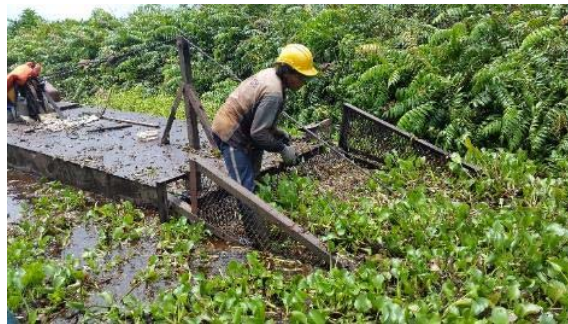
Figure 8 Canal Cleaning Using Mechanical Equipment "Bulldozer Lumut"
