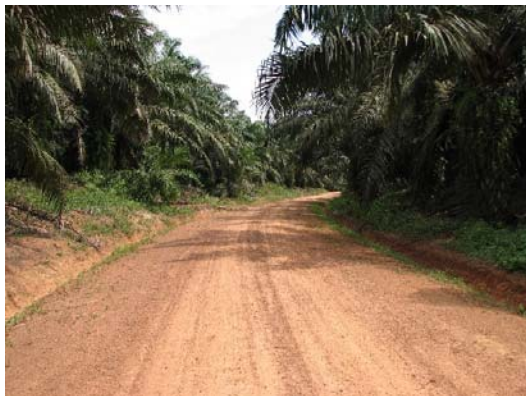
Plate 4: Well Maintained Smallholder Access Road
