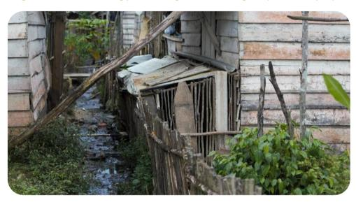
Figure 8 Photo showing poor drainage at the housing complex in Company C
