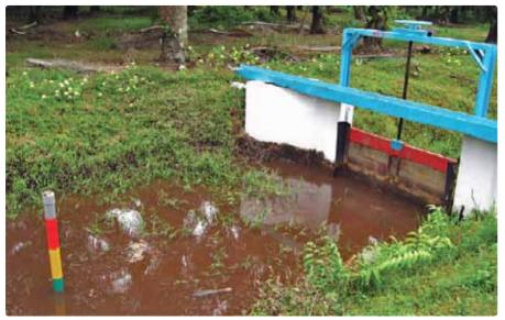
Figure 7-3: An example of a water control structure.
