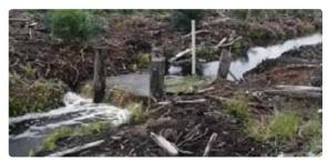
Figure 3-4: Water control structures do not need to be expensive structures and can be simply constructed with wood or sand bags.
