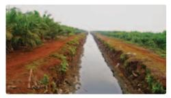
Figure 3-8: Over-drainage in main drain in a peat dome area during dry seasons may result in high CO<sub>2</sub> emissions, subsidence rates, increased risk of accidental fires, as well as significantly reduced yields.
