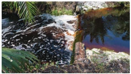
Figure 7-4: One weir installed at every 20 cm drop in water level to enable water retention along collection drains.
