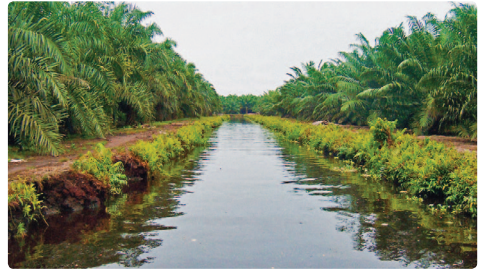
Figure 3-7: Optimal water level management at 40-60 cm (in collection drain) results in a yield potential of 25-30 ton FFB/ha/yr.
