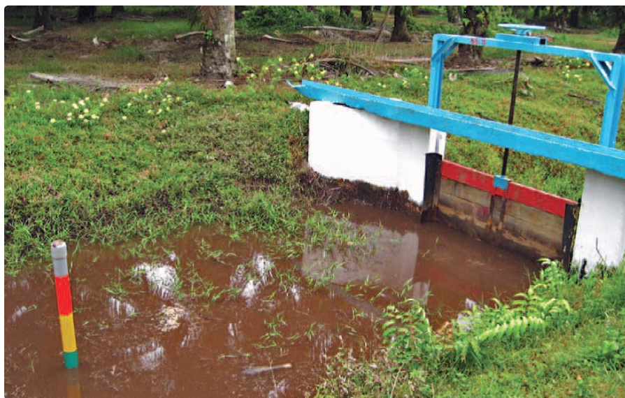
Figure 7-3: An example of a water control structure.
