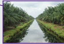
Branch Canal: 406 km, 6 m x 3 m
