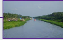
Main Canal: 21 km, 20 m x 5 m
