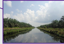
Collection Canal: 60 km, 12 m x 4 m
