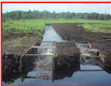
Figure 3-21: Water control structures.
