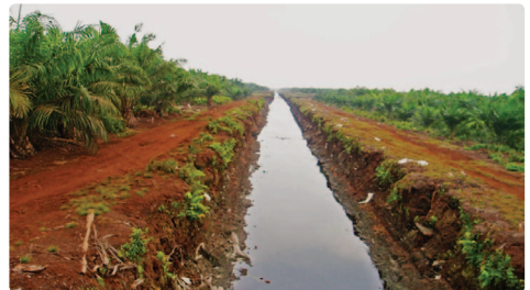
Figure 3-8: Over-drainage in main drain in a peat dome area during dry seasons may result in high CO 2 emissions, subsidence rates, increased risk of accidental fires, as well as significantly reduced yields.
