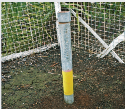
Figure 7-2: Photo in 2010 of a subsidence pole installed in late 2007, 10 years after initial drainage.
