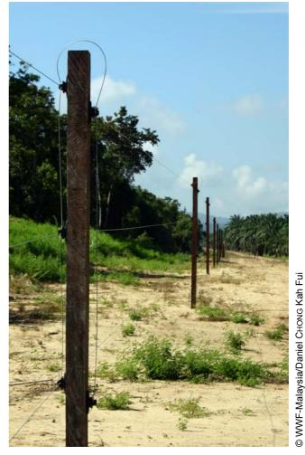
Figure 6. A three-strand electric fence with the posts wired.
