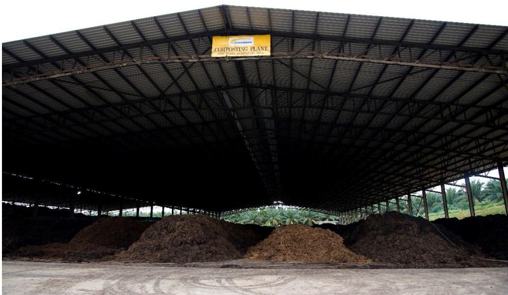
Figure 52. Composting Facility at Sime Darby's mill
