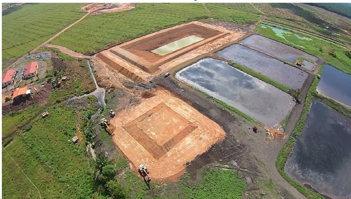
Figure 46. Aerial View of Methane Capture and Biogas Plant Site during Construction
