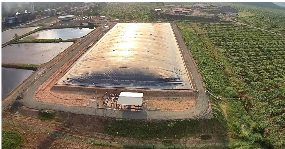
Figure 41. Methane Capture Facility at Terusan Mill
