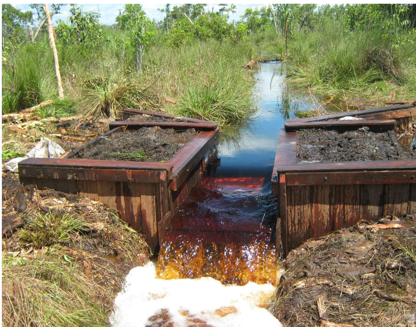
Figure 18. Examples of a box dam to rewet degraded tropical peatland forest (source: WWF)
