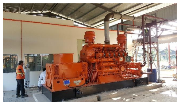
Figure 47. Left: Construction of lagoon, Right: Biogas engine
