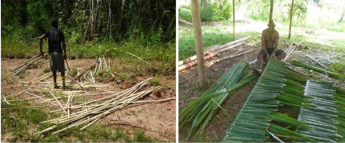
Figure 12: Construction of sago thatch roofing panels. Left image, Pandanus spp 'batons' being split for thatching supports, and right image, sewing sago thatching
