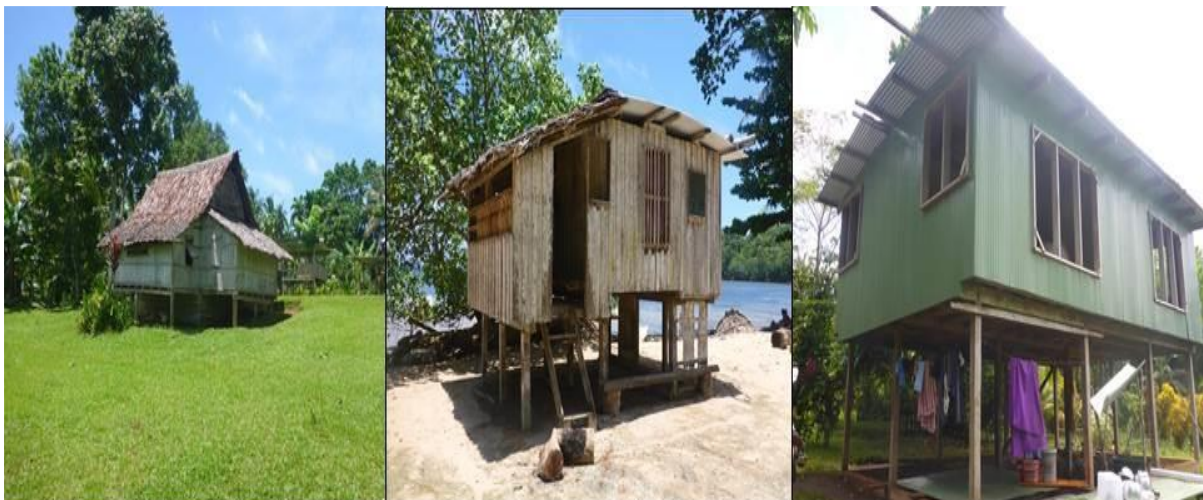
Figure 11: Common housing construction materials in Lokono Village. Left image, ‘bush’ material construction, middle image, mixed ‘bush’ and ‘modern’ material construction and right image, ‘modern’ material construction
