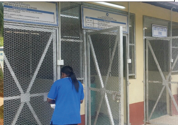
Chemicals store and Scheduled Waste store at Gomali Estate.
