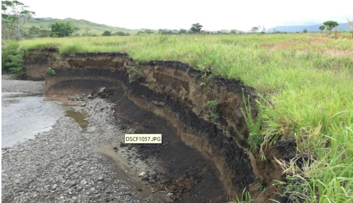
Figure 4 Cross-sectional profile of shallow loam soil – eroded inner bank of Beboi Creek
