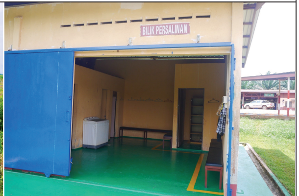
Bukit Paloh estate: Showering and washing facilities for the field workers.
