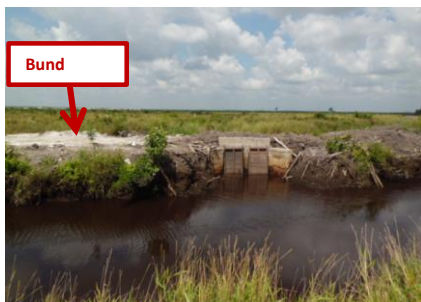
Figure 4. System with Bund and Flap Gates. The Flap Gates closes automatically during high tide, preventing influx of tidal water (Left). The Flap Gates open automatically during low tide, allowing drainage (Right).
