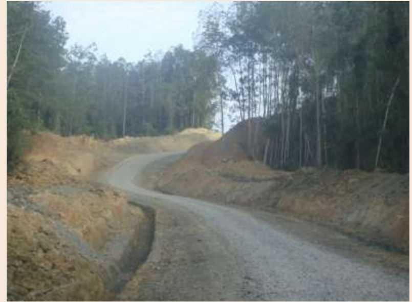
Current condition of timber road from Rh Iba to Keresia Plantations(17km)
